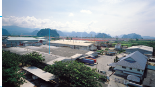
Rubberex Manufacturing Complex
