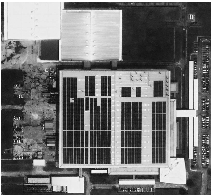
A 2.30 megawatt peak solar PV system installed at an industrial building in Subang Jaya, Selangor
