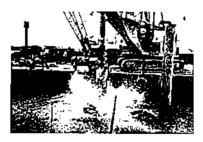
Marine pre-bore and piling works are required prior to the construction of water structures such as jetties, bridges, ports and water chalets.
