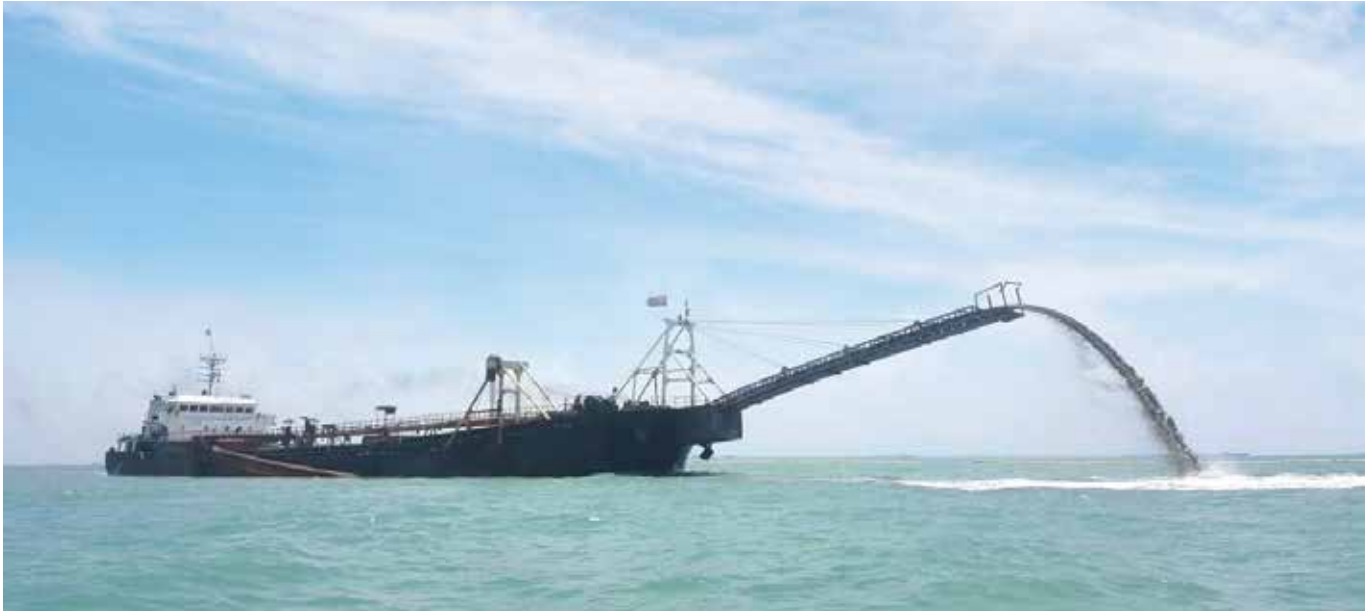
Sand discharging operation.
