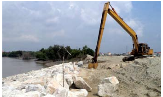
• Earthwork, River Protection and Associated Works at Glenmarie Cove, Klang, Selangor
