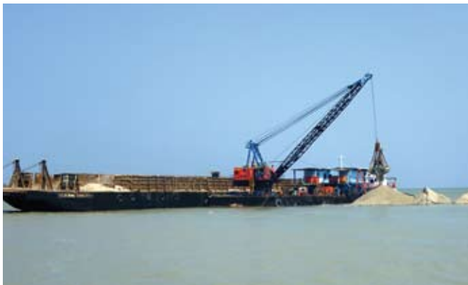
• Reclamation Works at Melaka
