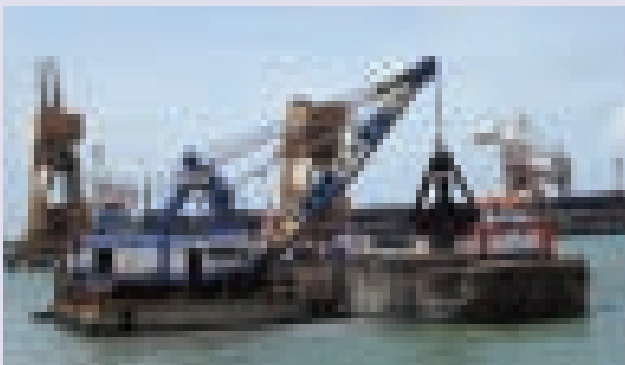
Maintenance Dredging at Stesen Janaelektrik Sultan Salahuddin Abdul Aziz, Kapar, Selangor
