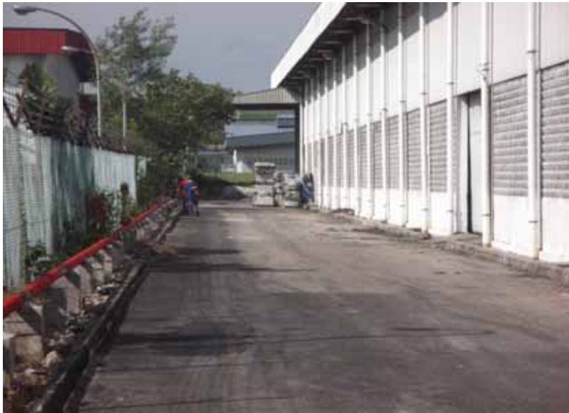
New resurfaced driveway.
