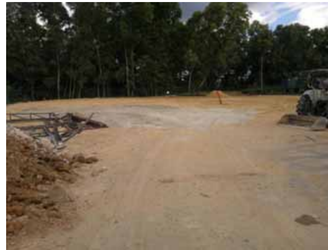
New Car Park – crusher run completed
