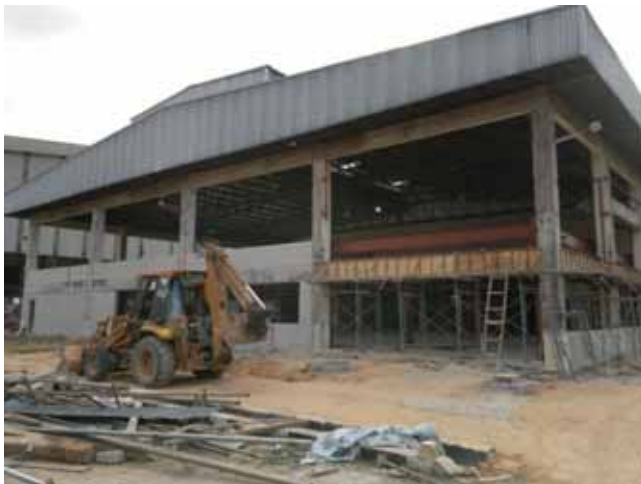
External View – Facing Car Park
