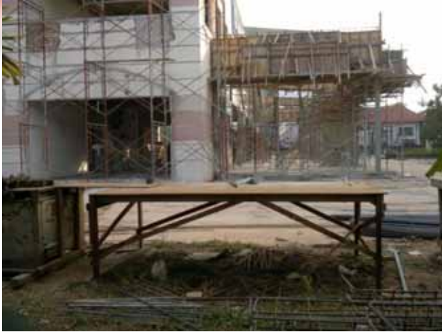
Main Lobby Construction
