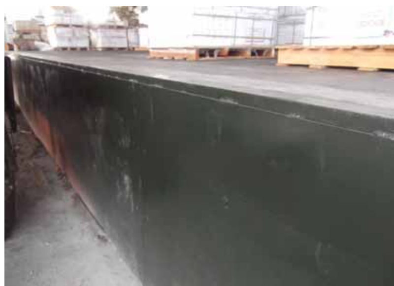
New protective mild steel plate installed for the Loading Bay
