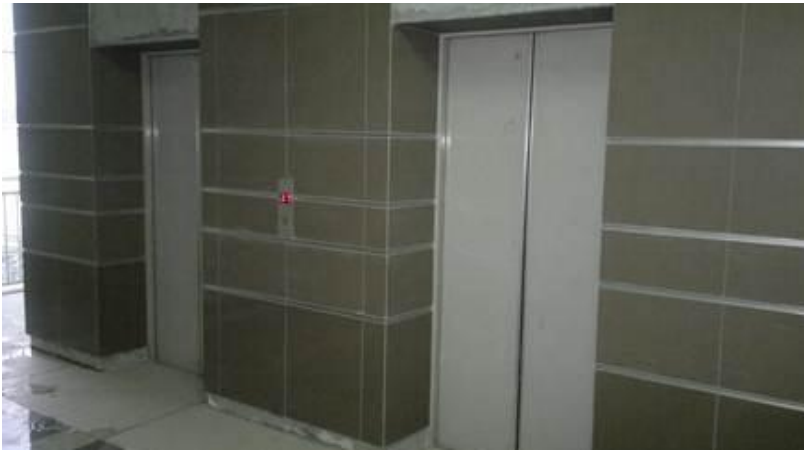
Third floor lobby new wall tiles
