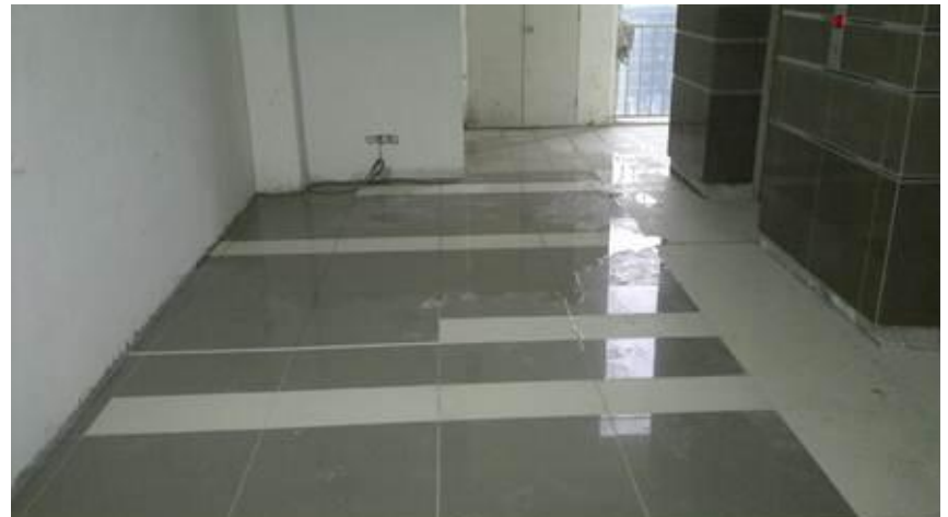
Third floor lobby in new tiles
