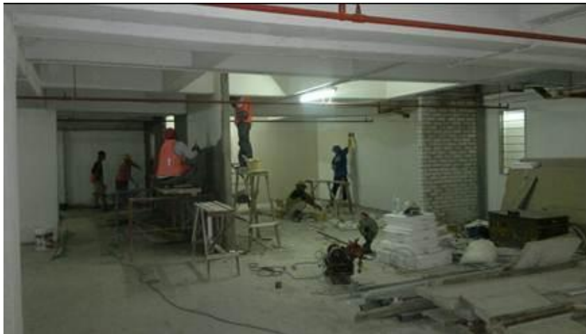
New Gen-Set room in construction
