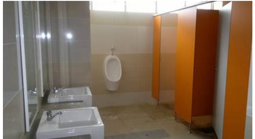
Male toilet at First floor
