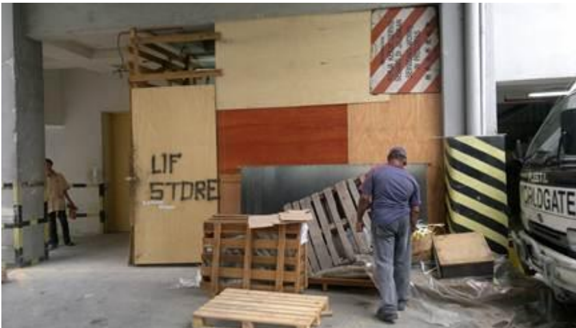
New Cargo lift installation
