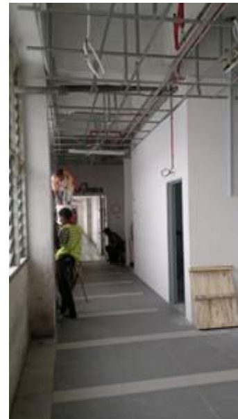
Third floor warehouse new corridor works in progress
