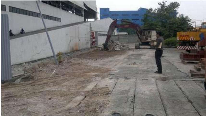
Phase 1: Sub-station piling works in progress
