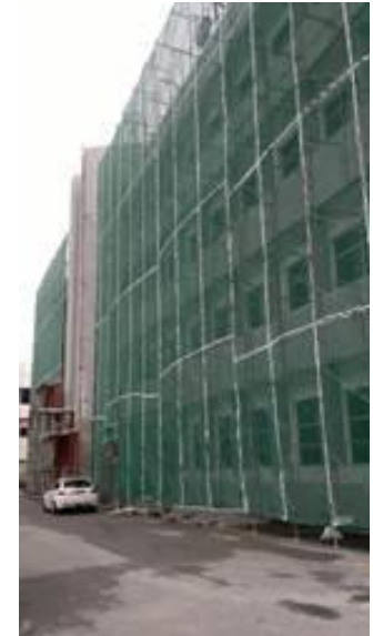
Scaffolding erected for new cladding
