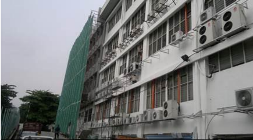
A/C relocation in progress
