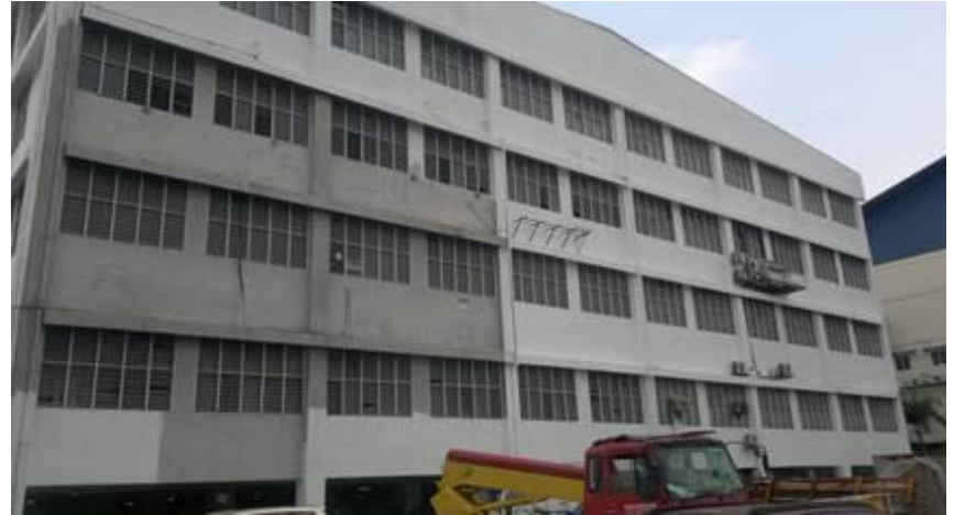
External painting in progress
