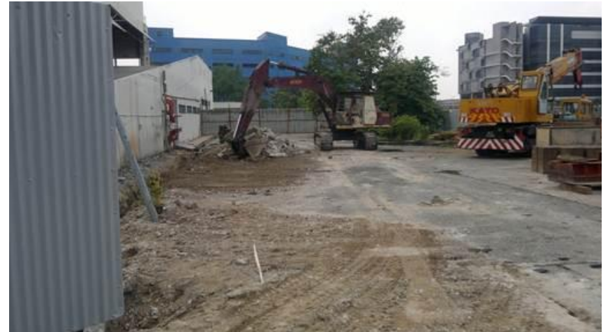
Phase 1: Sub-station piling works in progress
