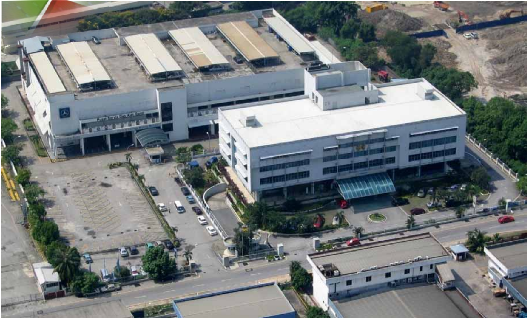
Current Building Complex
