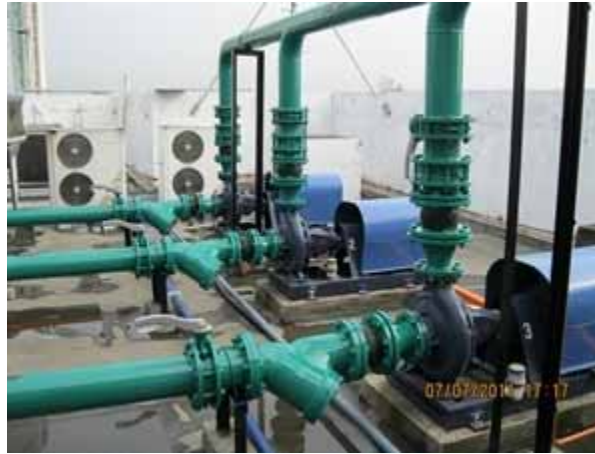
6 new pumps installed
