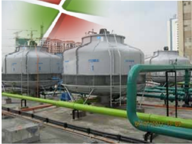
6 new Cooling Towers Installed
