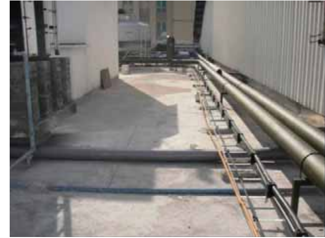
New waterproofing installed
