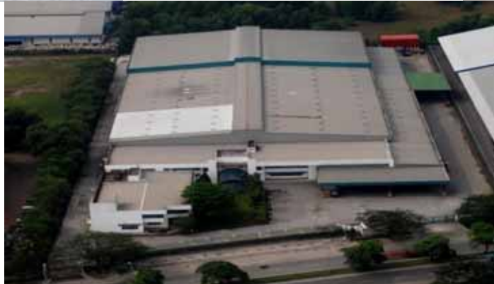
North Port Logistics Centre 1, Klang
