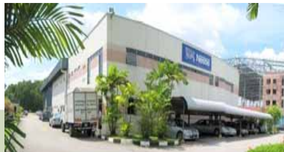
Nestle Office & Warehouse, Shah Alam
