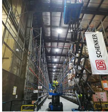
Seberang Prai Logistics Warehouse 3 Upgrading of warehouse lighting to LED lighting
