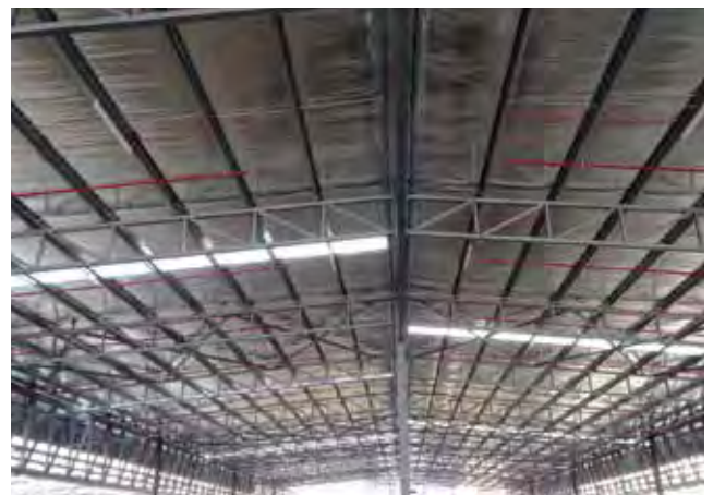
Completed roof structure with fire fighting system
