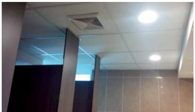
New LED lights with motion sensor
