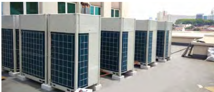
New VRV air-conditioning system
