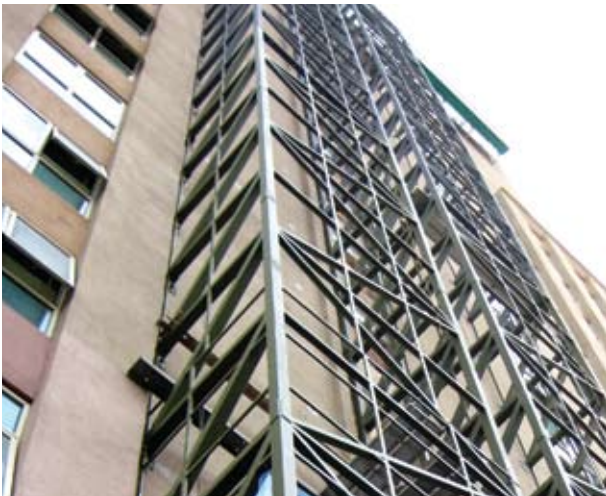
External lift skeletons being installed
