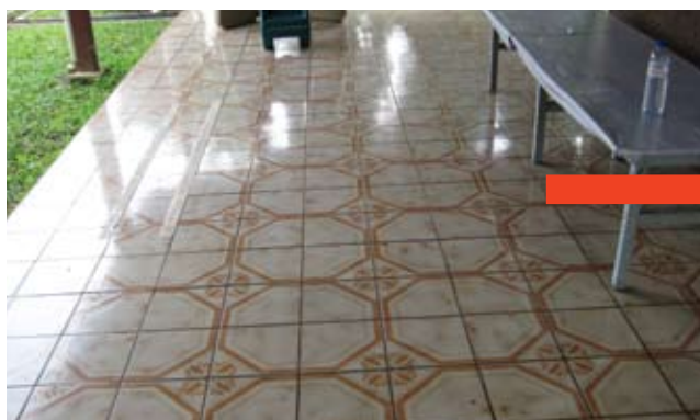
Slippery tiles caused accidents and were replaced by new non-slip homogenous tiles
