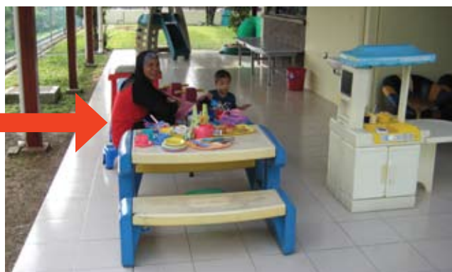
Slippery tiles caused accidents and were replaced by new non-slip homogenous tiles
