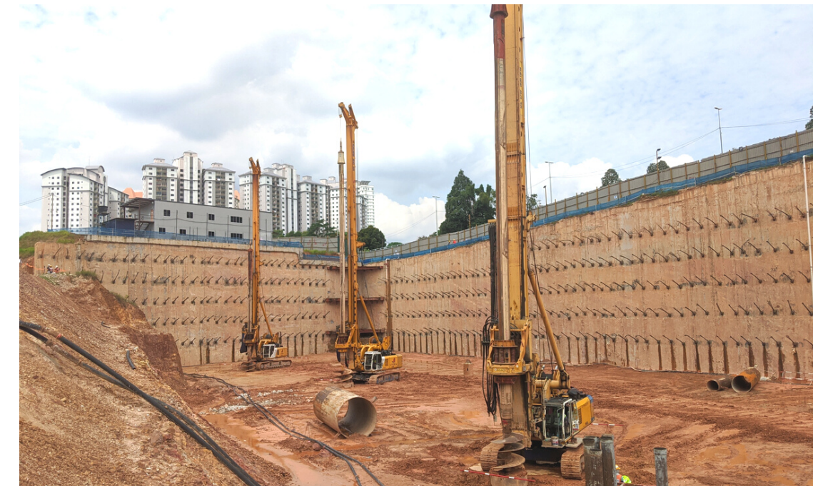
German-grade Rotary Drilling Rigs MET5 @ KL Metropolis Project
