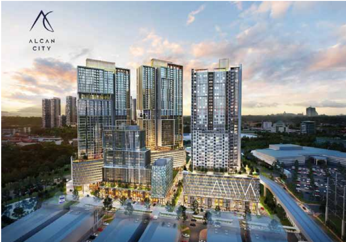
Artist's Impression of Alcan City in Bandar Baru Klang: A Glimpse into the Development's Innovative Design and Modern Aesthetic
