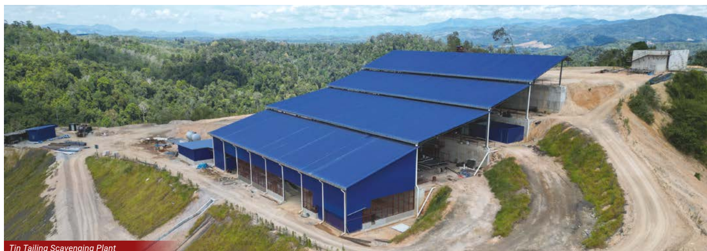
Tin Tailing Scavenging Plant
