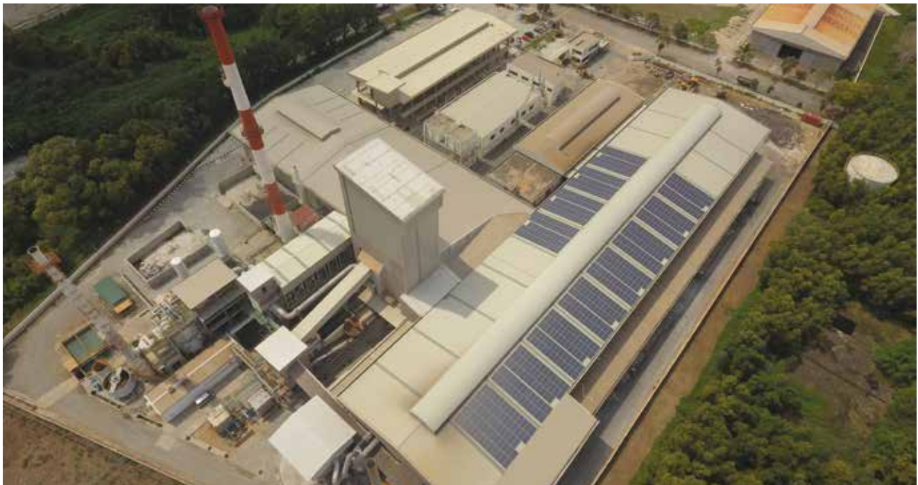
→ Solar PV panels at Pulau Indah smelter
