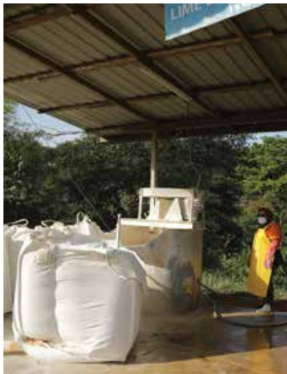
→ Lime dosing operations
