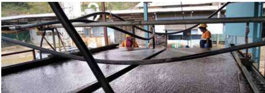
→ Mechanisation of operations for increased efficiency
