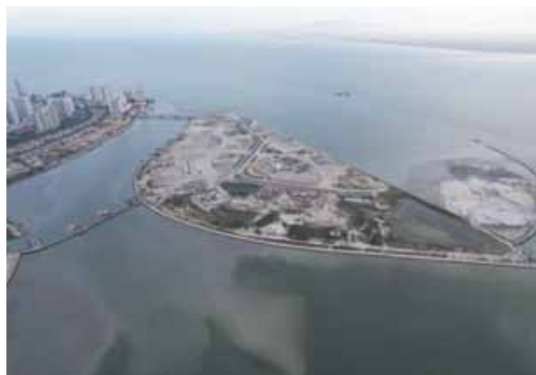
Dredging & Rock Bund
