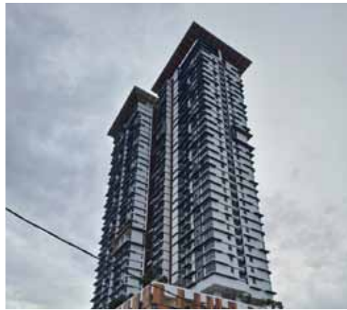
Megah Rise Mix Development @ Petaling Jaya
