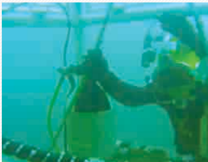
• Underwater work in action
