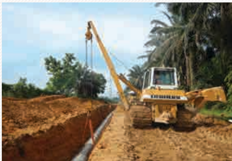
• Pengerang Project - Line pipes lowering into trenches
