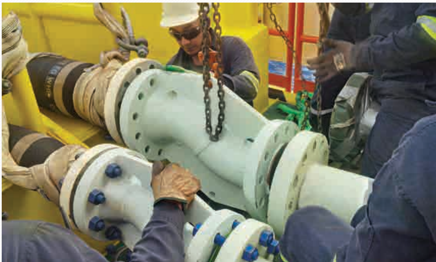
• Goose-neck pipe joints installation at Bertam-A Platform for Lundin Petroleum
