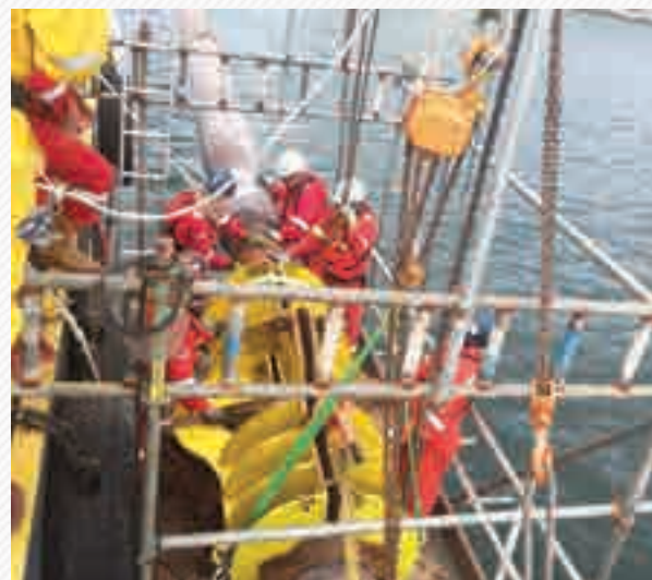
• Pipeline installation in Dalak, Sabah
