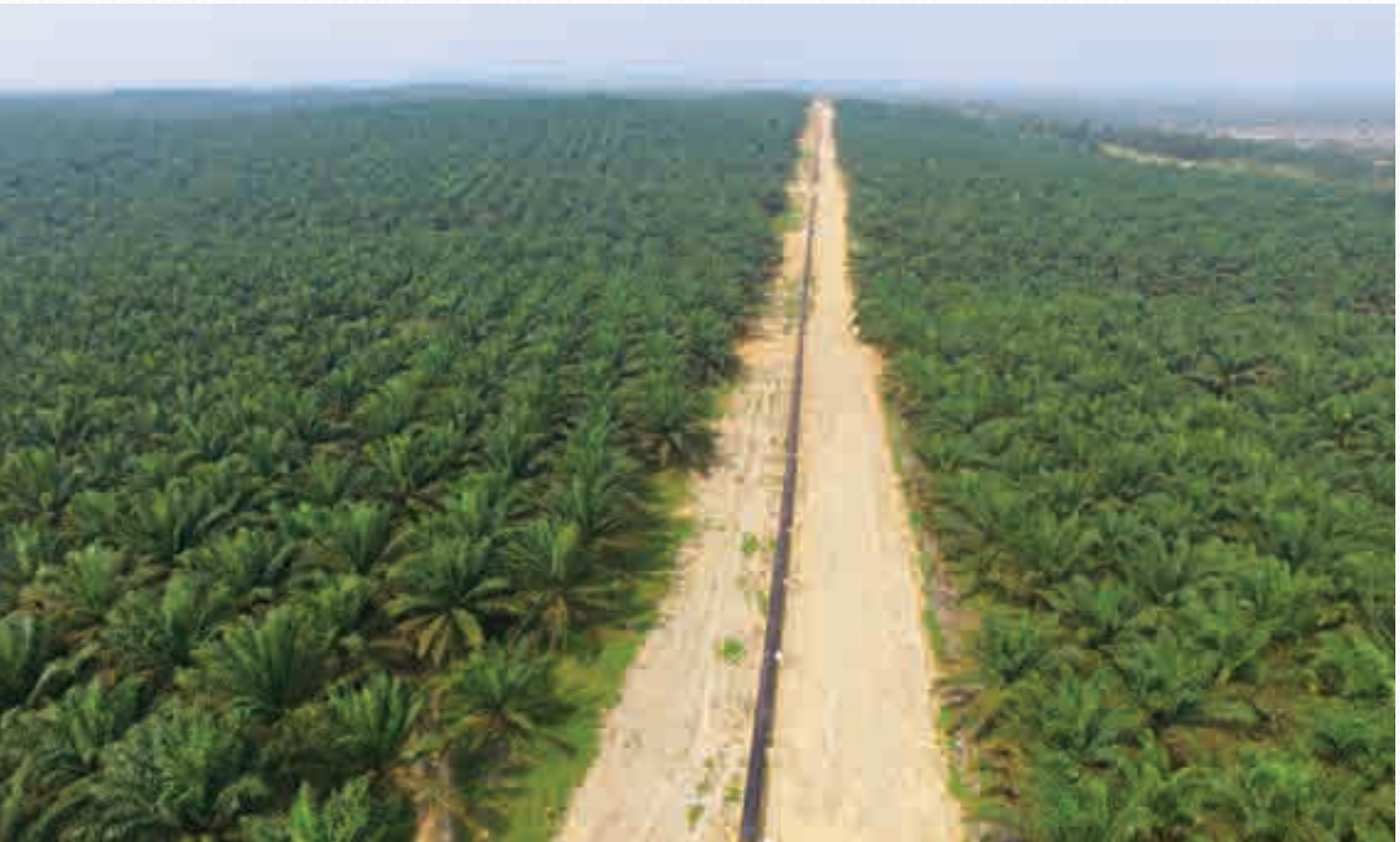
• Pengerang Project - Aerial view of part of 73km pipeline
