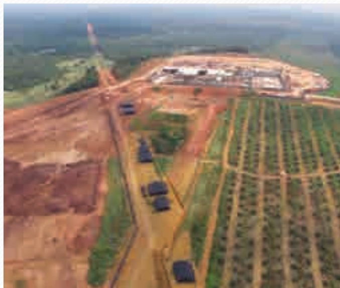
• Pengerang Project - Line pipes awaiting to be stringed
