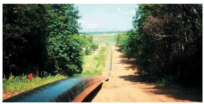
■ EPCC Prai Lateral Pipeline - Stringing of line pipes
