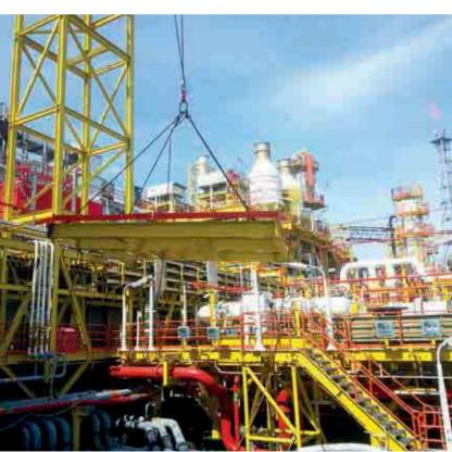
■ Lifting structure panel for dual fuel skid at Cendor FPSO
