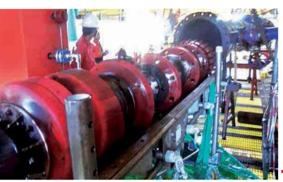
Loading of an intelligent pipeline inspection gauges
