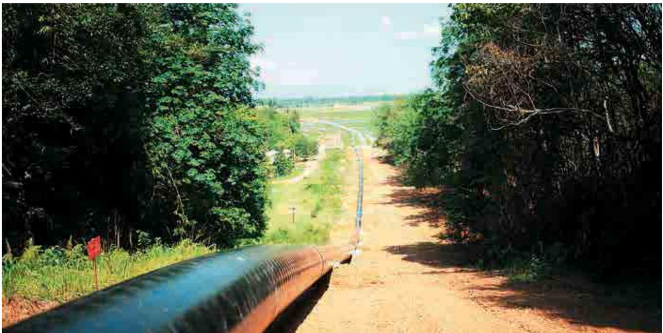
■ EPCC Prai Lateral Pipeline – Stringing of line pipes
