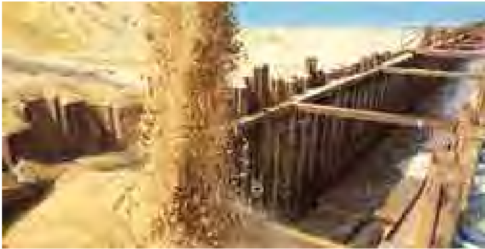
Construction of Cofferdam
